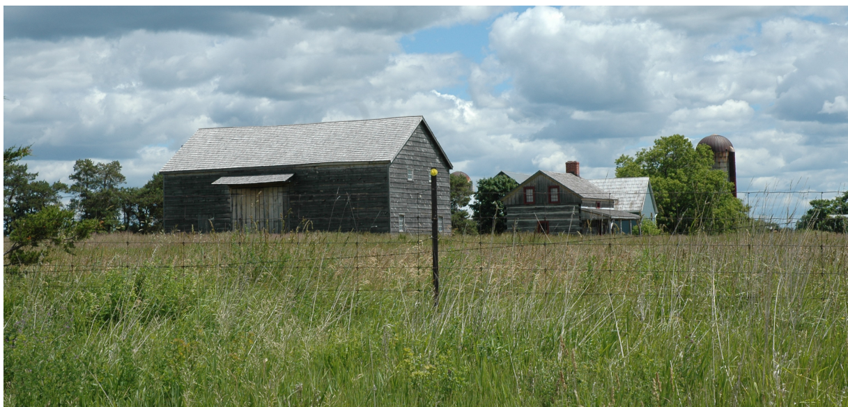
Plate 5 The Gibbins' Property, view from Dainard Road facing northeast
