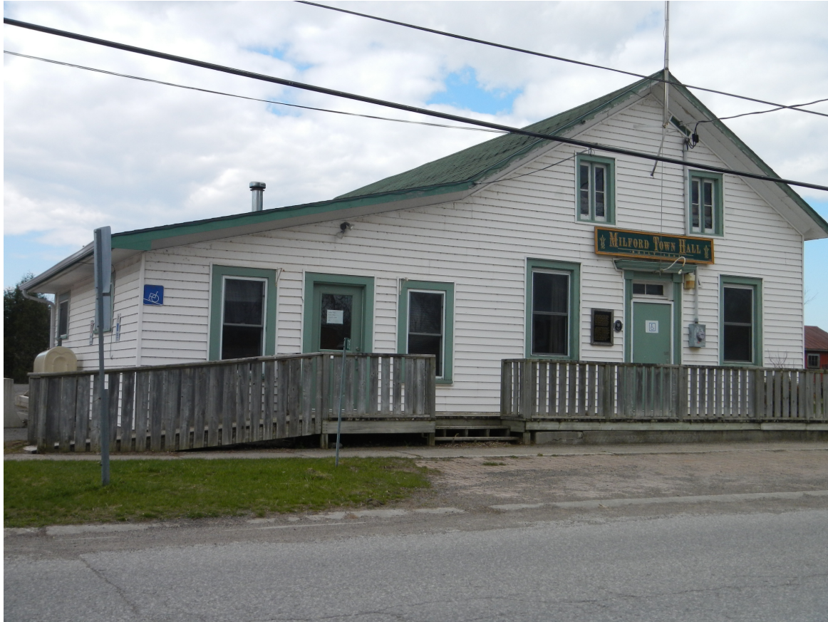
Plate 6 Milford Town Hall
