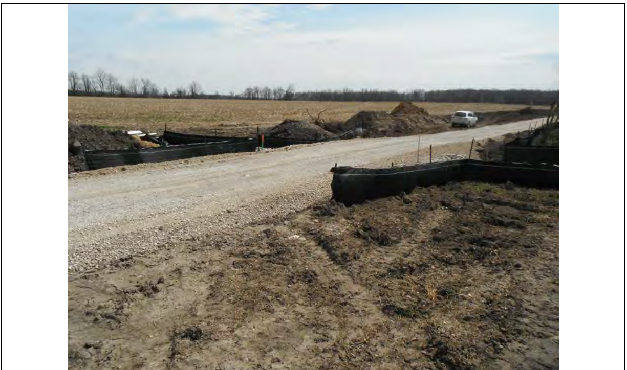
Photo 2 Typical access road construction at a wind project
