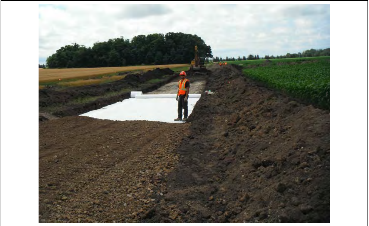
Photo 5 Typical access road construction at a wind project
