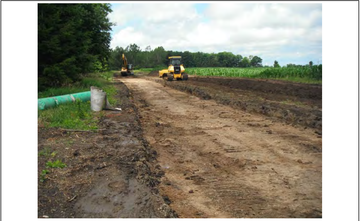
Photo 3 Typical access road construction at a wind project
