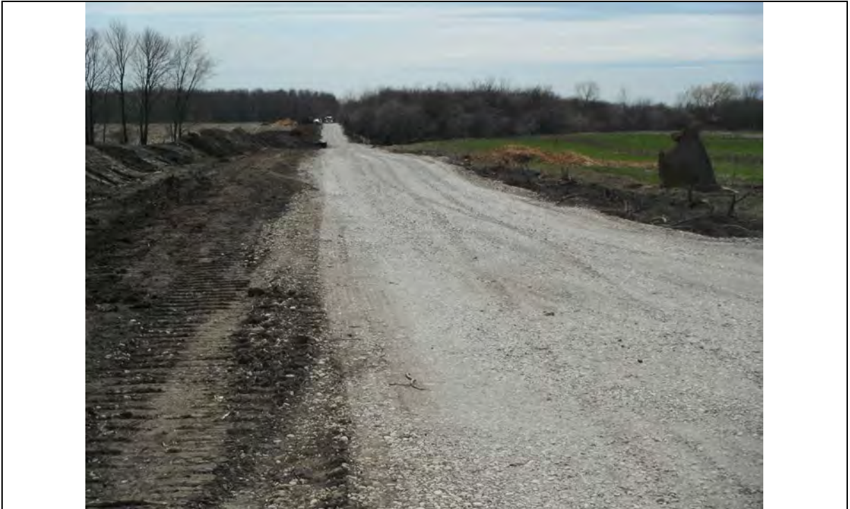
Photo 1 Typical access road construction at a wind project
